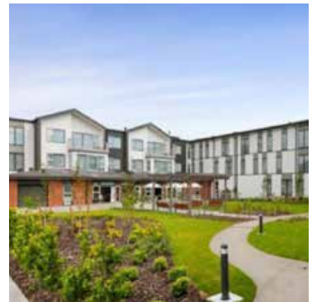
BUPA RETIREMENT VILLAGES NAPIER, TOTARA, CROFTON DOWNS, PALMERSTON NORTH, ASHFIELD
