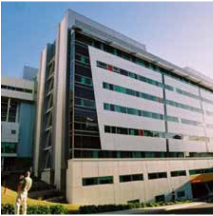
AUCKLAND HOSPITAL AUCKLAND, NEW ZEALAND
